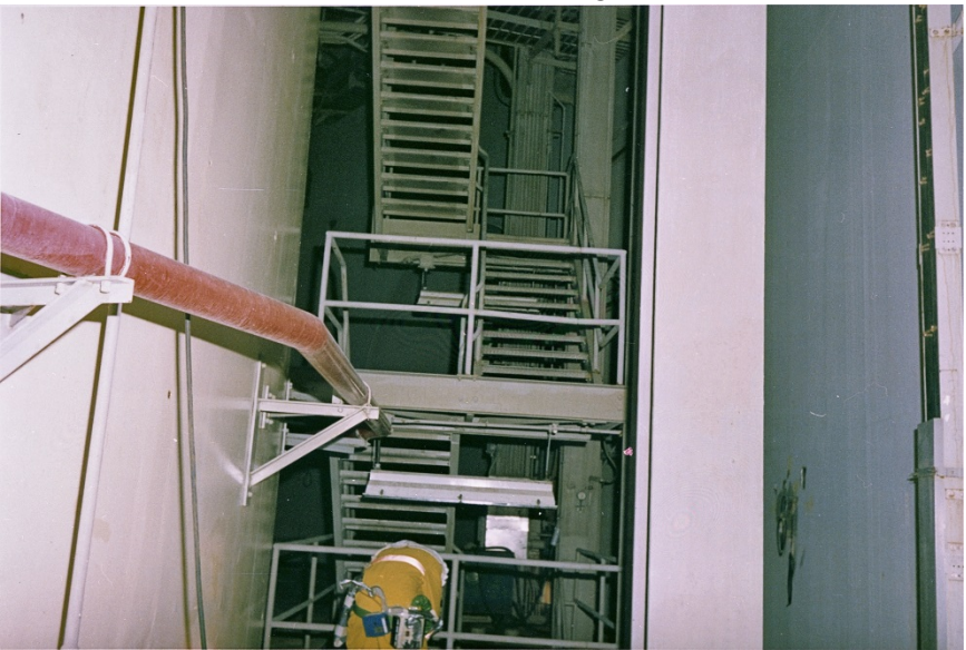
A technician lowering a telescoping radiation detector down into the open stairwell to the reactor building basement. Measurements revealed radiation levels of 40 to 45 rem per hour at 5 to 7 feet from the surface of water.
