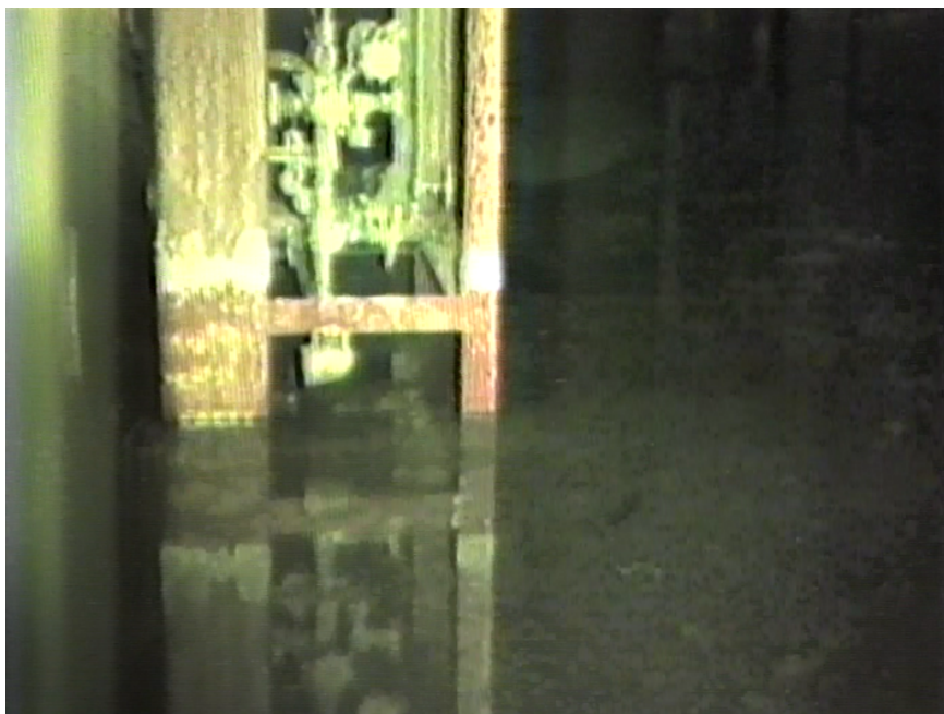
The basement in the reactor building contained about 8 feet of highly contaminated water. The submerged demineralizer system started processing basement water on September 9, 1981.
