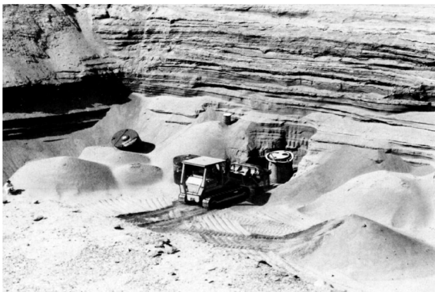
Demonstration high integrity container (HIC) being covered in the trench at the commercial radioactive waste disposal site near Richland, Washington. The HIC contained the highly loaded EPICOR II prefilter No. 18. The demonstration set the precedent for disposing of the remaining EPICOR II prefilters that were temporarily stored at INEL.
