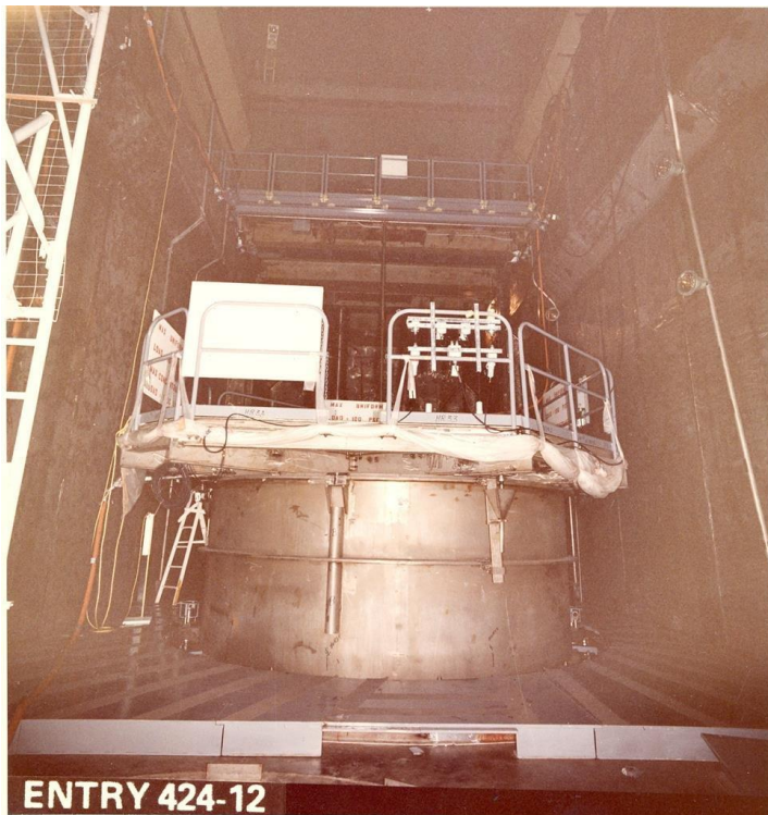
Internals indexing fixture with its temporary cover mounted on the reactor vessel flange. This fixture would eventually be mated to the defueling work platform.
