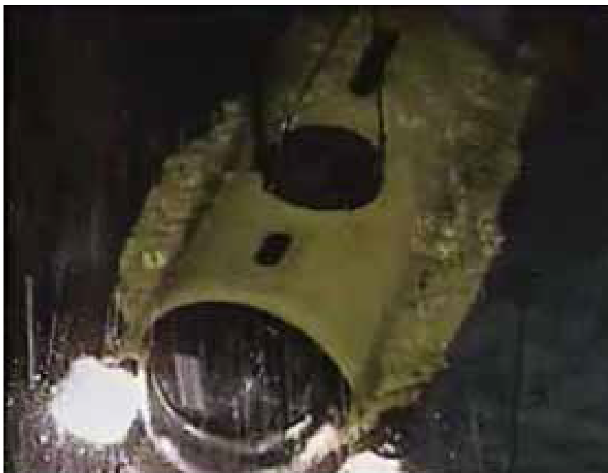
Remotely operated submersible vehicle equipped with an articulating claw and a scoop was used to remove larger pieces of debris that were located on the bottom head of the pressurizer.
