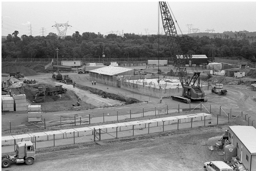
Solid waste staging facility was constructed to temporarily store radioactive wastes, such as dewatered resins, prior to shipment. Two module structures were built (center). The crane is loading a spent liner in a shipping cask. The temporary interim liner staging modules shown along the bottom.
