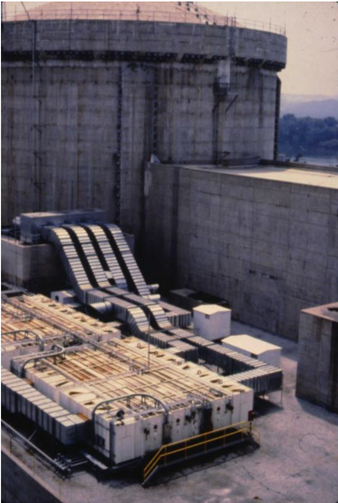
Temporary filtration system for the auxiliary and fuel handling building installed on the auxiliary building roof. TMI-2 reactor building in the background; fuel handling building at center right.
