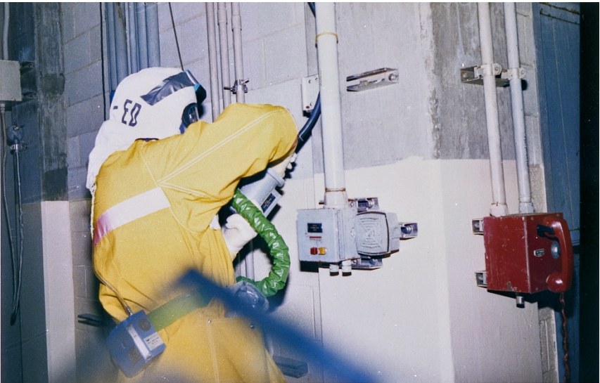
Several electrical components from the reactor building were retrieved and examined as part of the DOE-sponsored Instrumentation and Electrical Program. Shown is the removal of an area radiation monitor (HP-R-211) from the northeast elevator wall.
