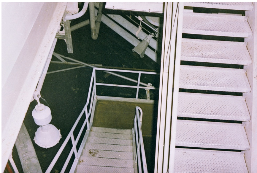
Water level in the basement reached the first stairwell landing indicating about 8 feet of water accumulation.
