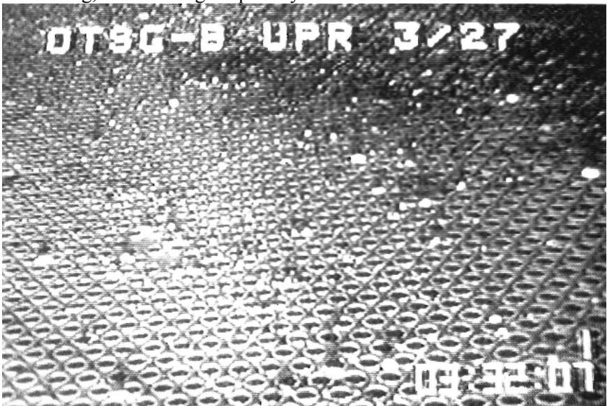
Fuel debris on the upper tube sheet of “B” steam generator.
