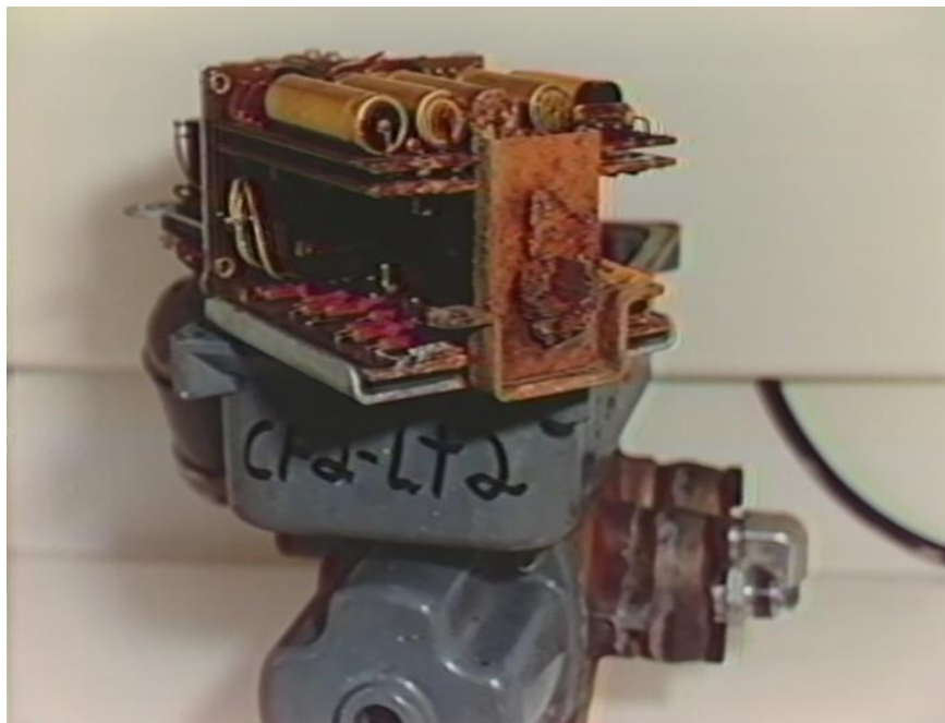
Core flood tank 1A level monitor CF-2-LT2 showing the condition of the enclosed electronic module. There was severe corrosion and degradation of internal components rendering the unit inoperable.
