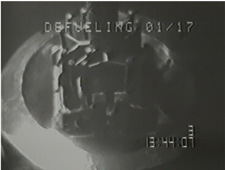
First loading of debris into a fuel canister started on January 12, 1986. Shown is an upper fitting of a control rod cluster being dropped into a
