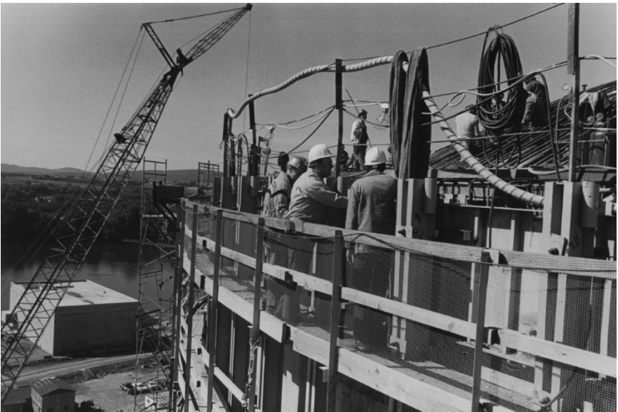
TMI-2 reactor building under construction. Shown is the top dome of the reactor building. The Susquehanna River can be seen in the background.
