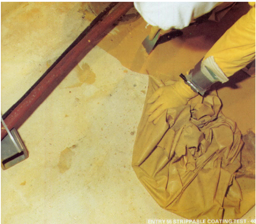
Strippable coating used in decontamination of floor surfaces.
