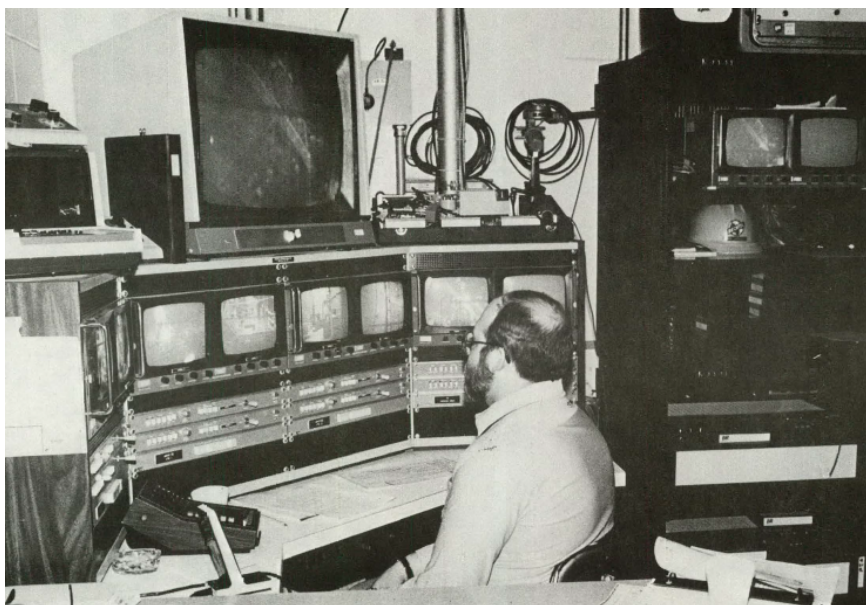
The command center for the gross decontamination experiment in March 1982 contained the control functions for entry into the reactor building with positions for safety, radiological engineering, operations, entry coordinator, and command center management.
