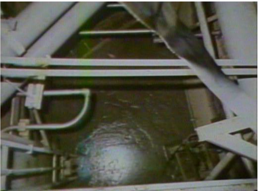
Highly radioactive sludge on the basement floor of the reactor building as viewed from an upper level. A robotic desludging system was used to vacuum the 40 percent of the basement floor area that was accessible to the robot.
