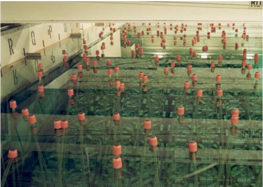
Above: The Model 125-B shipping cask being removed from the rail car at the Central Facilities Area at INEL. Both impact limiters are shown removed from the ends of the cask. Below: Defueling canisters in the temporary storage pool at INEL. A vent tube was installed on each canister for continuous venting.
