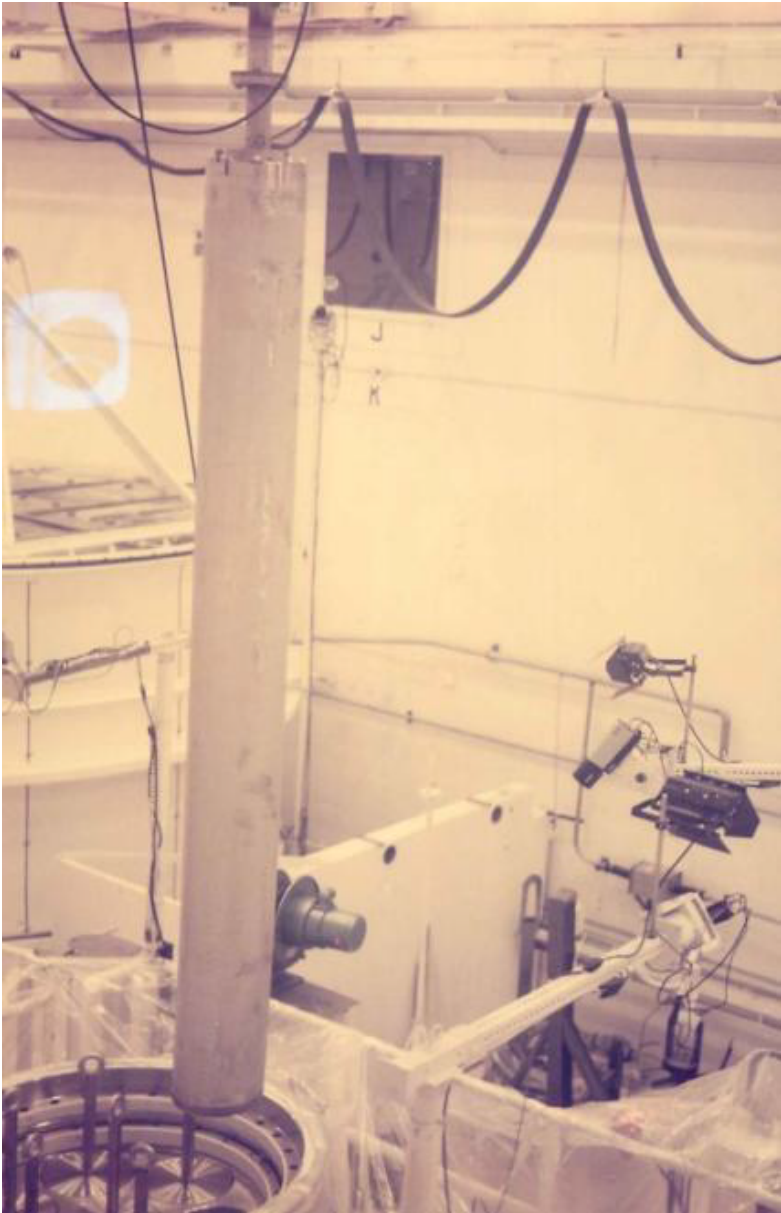
A loaded defueling canister being remotely lifted from the shipping cask at the INEL receiving facility. The 12.5-foot long canister was filled with water, placed in a storage module, and transferred to the storage pool for temporary storage at the INEL.
