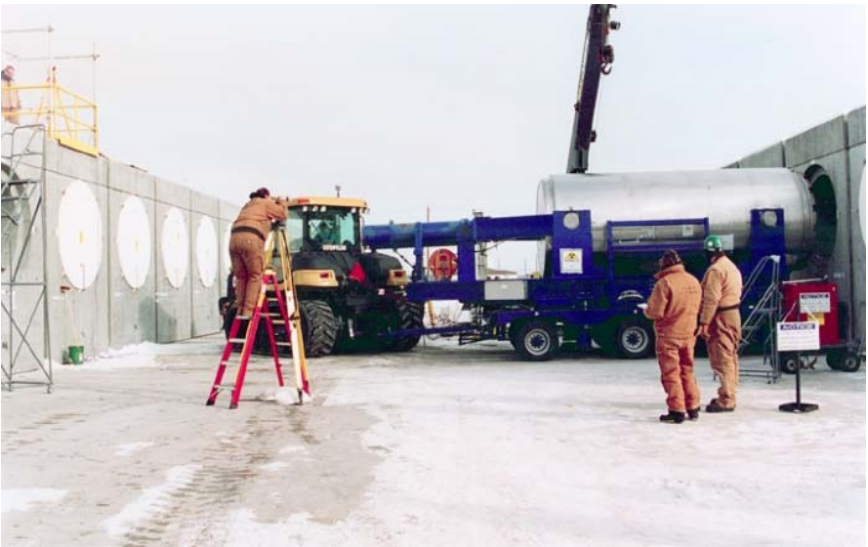
Independent spent fuel storage installation (ISFSI) for the dry storage of TMI-2 fuel debris located at the INEL. The TMI-2 defueling canisters were removed from the storage pool, dewatered, dried, and placed in a dry shielded canister. The dry shielded canister with up to 12 defueling canisters was placed inside a reinforced concrete horizontal storage module. The ISFSI was certified and licensed by the NRC.
