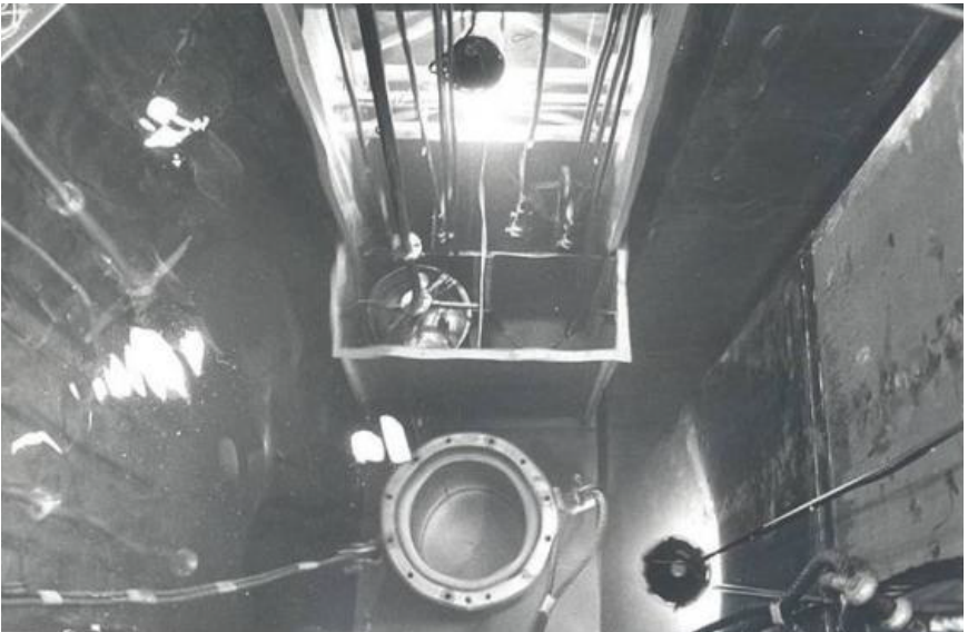
A highly radioactive spent SDS resin liner (center) being transferred into a shipping cask (lower center) while underwater in the spent fuel pool.
