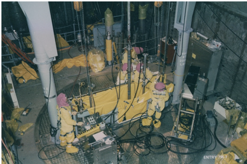
Defueling operations from the rotating defueling work platform with a worker holding a long-handled defueling tool down through the slit into the reactor vessel. Two jib cranes at each end of the slit were used to lower larger tools.
