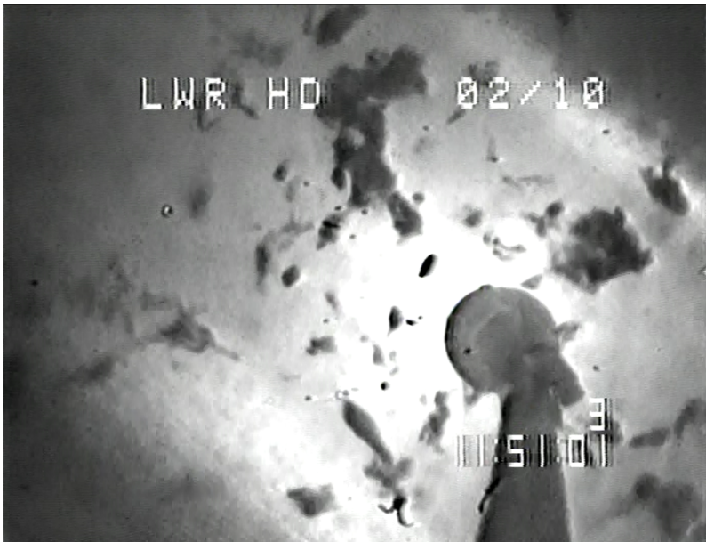
Problems plagued the cleanup systems early because of microorganism growth in the reactor coolant. The resulting loss of visibility halted all defueling operations for a few months. Shown is a view down into the reactor vessel annulus region between the core support assembly and the vessel wall. (A light hanging at the lower right.)
