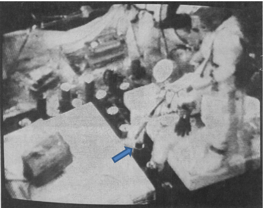
The first closed-circuit video inspection of the upper reactor core region was performed on July 21, 1982. A technician sitting on a platform positioned on top of the reactor vessel service structure is inserting a camera, 1.5 inches in diameter and 12 inches long, through an empty leadscrew support tube.
